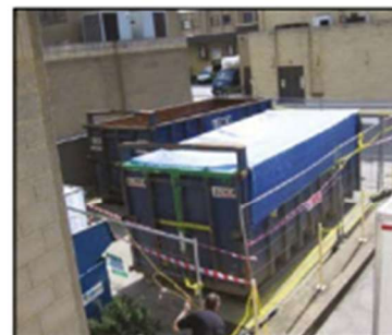
It is not good enough to throw sheeting over a standard skip
